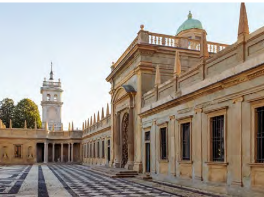
Above: the north facade of the neoclassical sandstone nymphaeum, with the white water tower seen in the distance. The tower contains a copper tank that can hold 1,980 US gallons of water, and this supplies all of the water features. Right: the Windmill Court is named after the fountain in the center, which includes a
